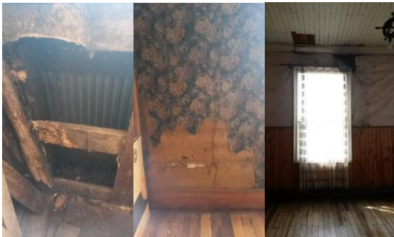
Figura 7: Interior muros (autor 2016)
