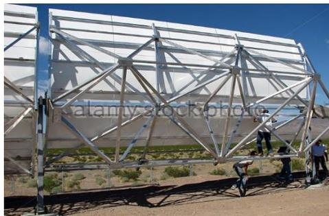
Figura 4.1: Estructura colector Solargenix [7]
