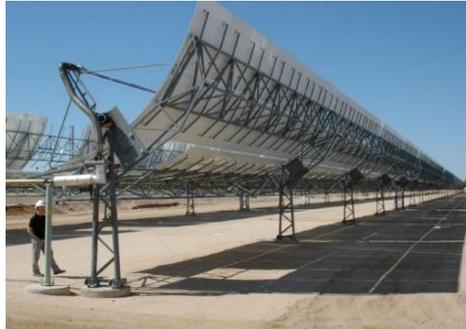
Figura 4.2: Filas colectores Eurotrough SKAL-ET [15]
