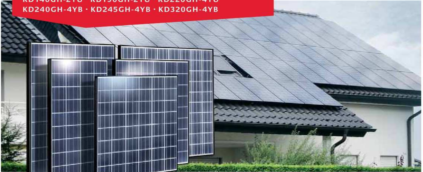
A partment house, Germany
