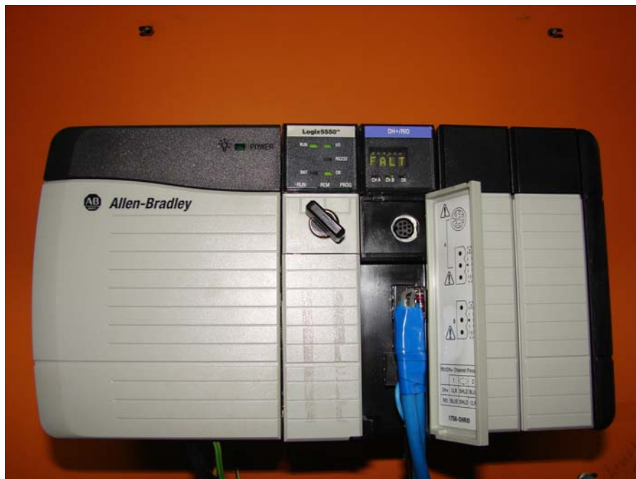
Fig. N°1: PLC ControlLogix 5550, Allen-Bradley
